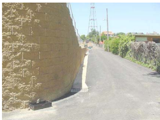
Figure 3.5. Textured blockwork on a curved wall that casts interesting shadows
