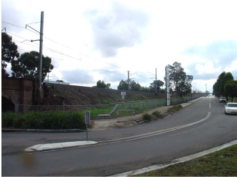
Figure 2.2 View of western side of Broomfield Street, near the underbridge
