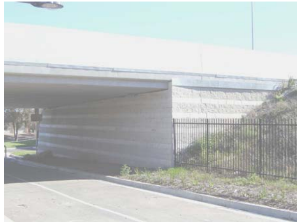
Figure 3.4. Underbridge wall with striped bands
