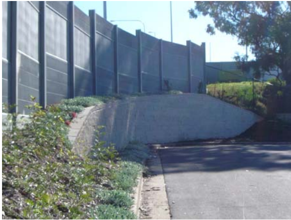
Figure 3.3. Retaining structure and noise barrier, with established planting
