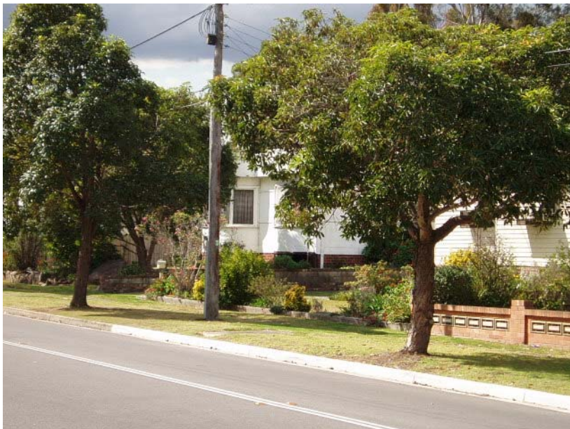
Figure 2.1. View of houses, eastern side of Broomfield Street
