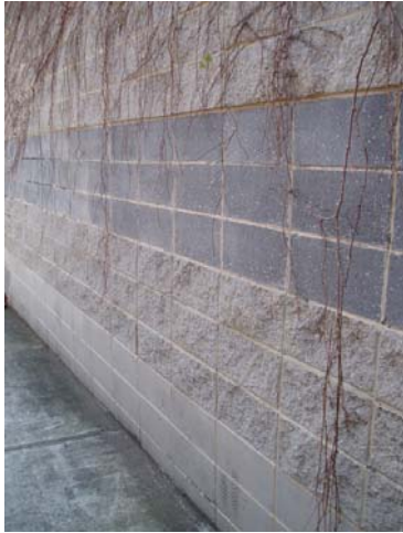
Figure 3.1. Blockwork noise barrier made up of textured and coloured panels
